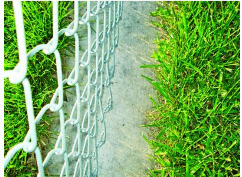
Concrete Mow Strip under Fence
